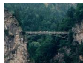
Marienbrücke Bridge as seen from the castle
